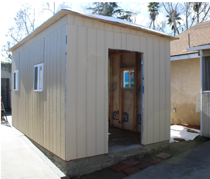
Building Under Construction
