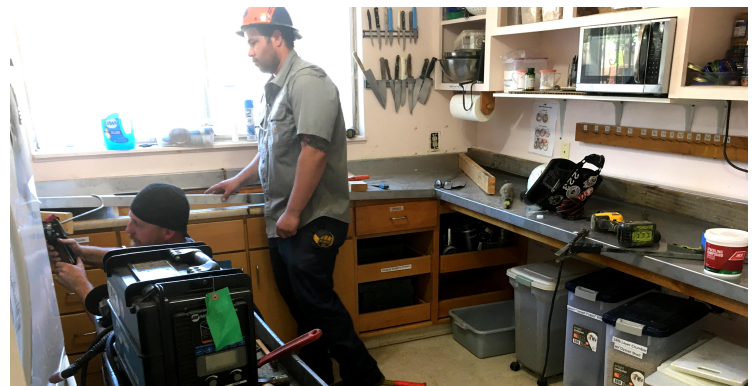
Installing the Kitchen Counters
