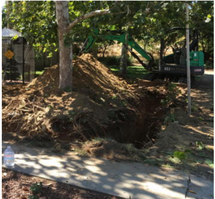
Leach Line Repair.
